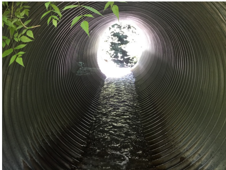
Looking through culvert from inlet
