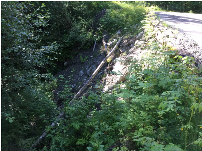
Downstream right approach fill slope
